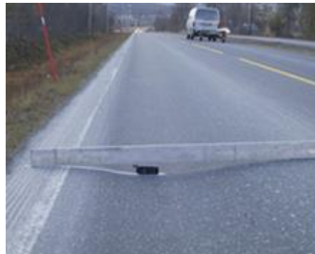
Figure 1. Rutting phenomenon occurrence in asphalt pavement
